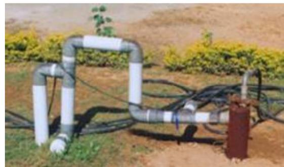
Bore Well Recharging by Roof Top Rain Water
